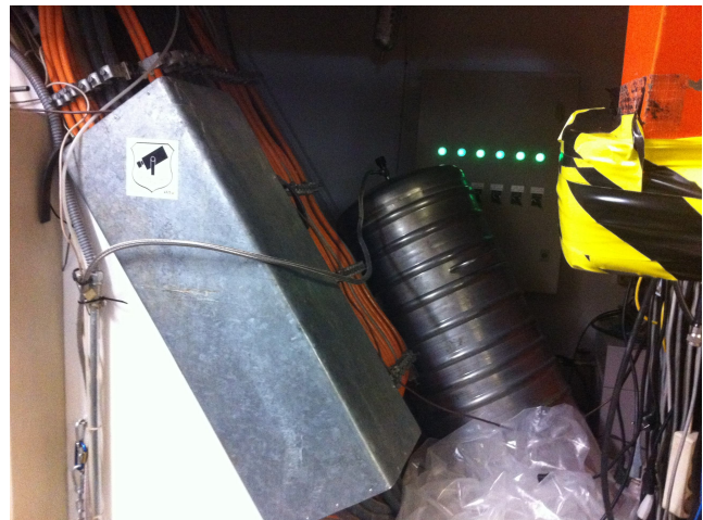
Picture 8: the Pulse Tube compressor and water cooling system location
